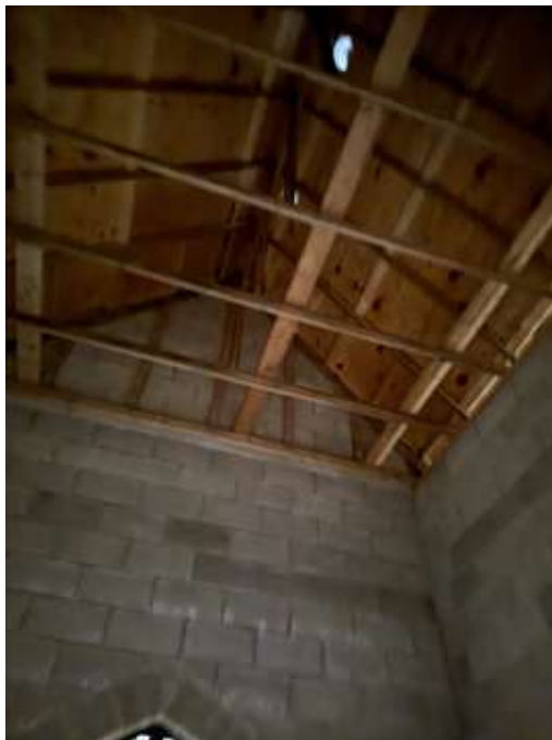
L: New pitched roof of bell tower
