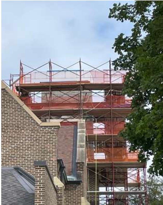
Northeast tower brick removed and new interior block being rebuilt. Taken July 20, 2025
