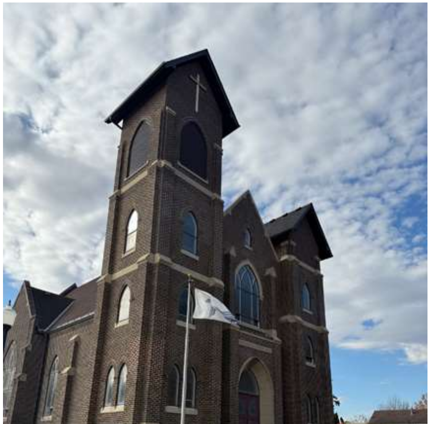
Towers with new pitched rooflines. New grates protect the interior of the bell tower from moisture but allow air filtration. Taken October 26, 2025
